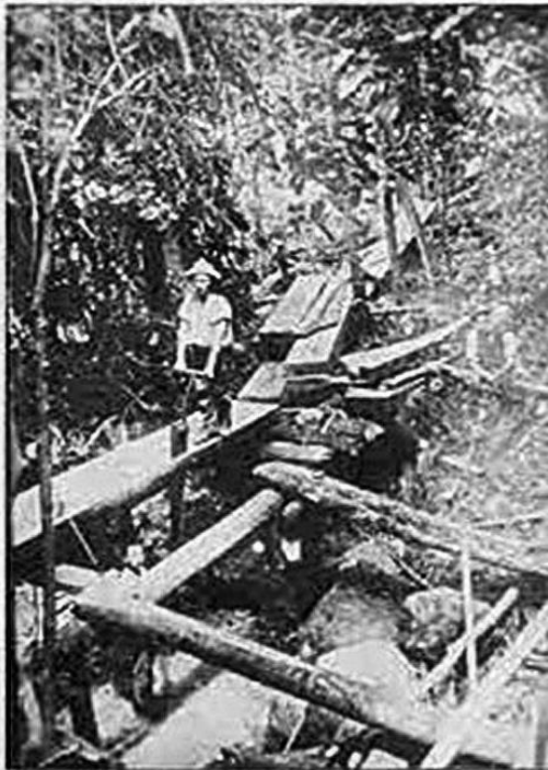
Early Timber Getters Using the Saw Pit Method with a Sawyer in the Pit Below
